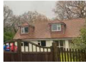
Figure 53: Pitched roof with red clay roof tiles and dormers.
