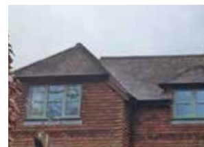
Figure 27: Half-hipped roof and corresponding pitch over a dormer window.
